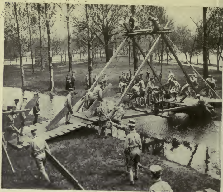
Building a Spar Bridge across a Stream twenty-seven feet wide— Culver
